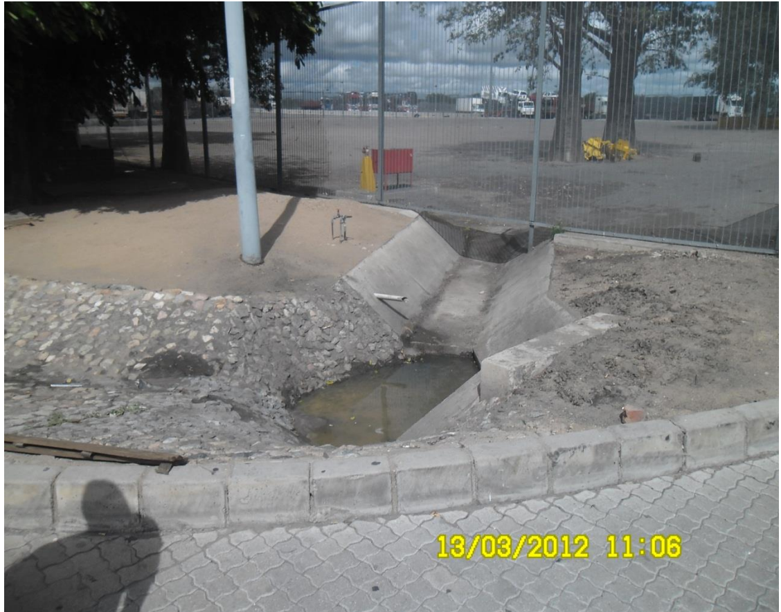
Figure 4-1 Trapezoidal channel discharging into the natural environment
